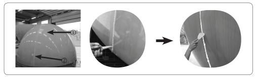
Spread Silicon between Radome Panels
